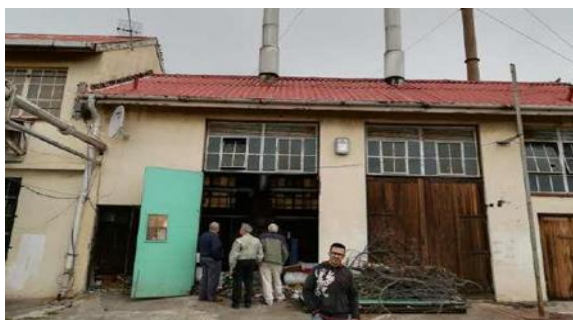
Photo 5: Azania Section- Former hospital incinerator
