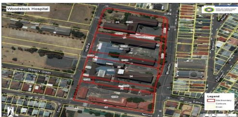
Photo 1 : Woodstock Hospital Site
